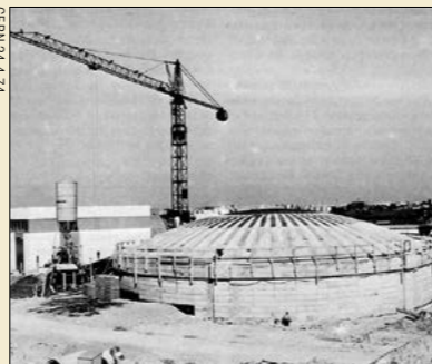
Two 5000 m 3 reservoirs are to hold the site water supply brought from Lac L man. One of them has already been filled and is distributing water to part of the site.
