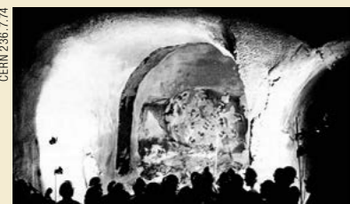
At precisely 10.32 a.m. on 31 July, the "mole" reached the end of its 7 km journey. A group of VIPs and journalists were present at the final breakthrough.
